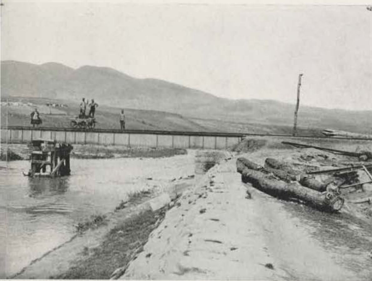
Line Belgrade-Nish-Vranje, 353 km. 004. Destroyed iron bridge of 40 and 20 metres opening over the Morava river.
