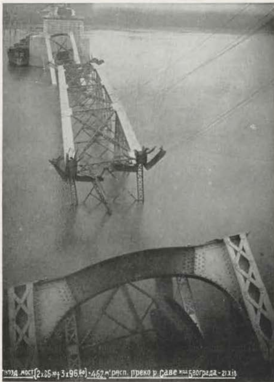
Railway line Belgrade-Zemoun-Budapest. Iron bridge on the river Sava of five sec- tions, with a total span of 462 metres.
